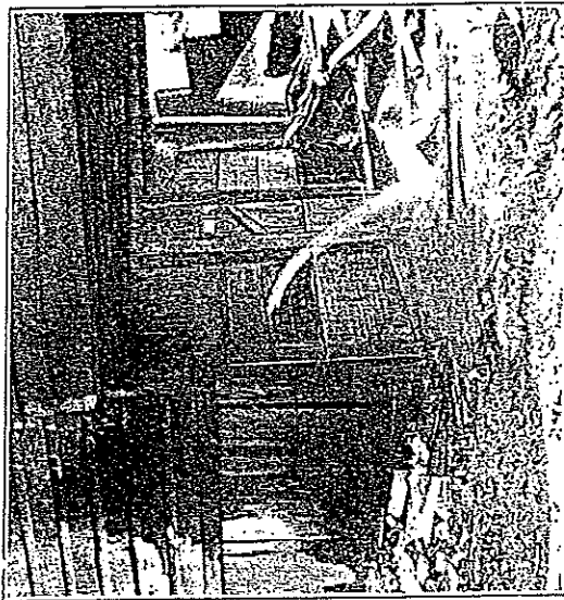
LANCASTER PIKE. House Drain Discharging. Water Flows Beneath House and Causes Stagnant Pool.
