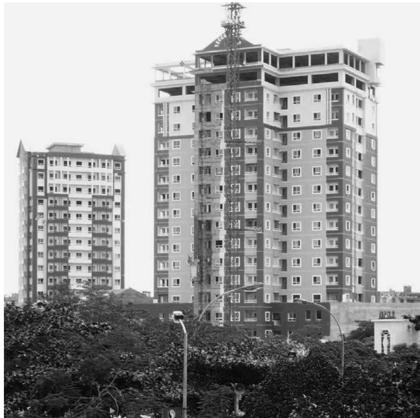
Figure 5 Quang Trung renovation, 2006. Photo by the author
