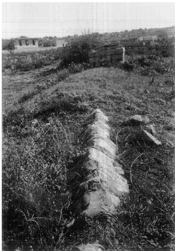
Figure 11.7. Galermi Aqueduct at Syracuse. Line of aqueduct channel, covered here by pointed roof, and leading to stone shaft in middle distance.
