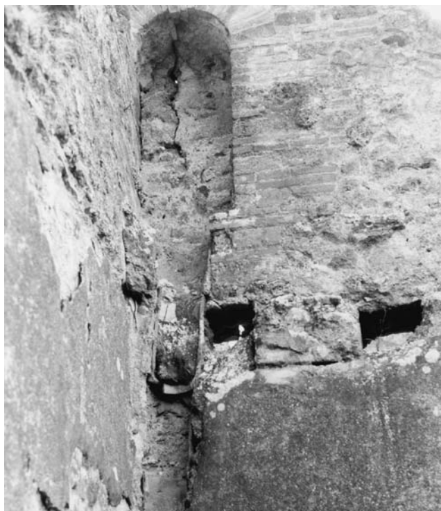
Figure 16.6 Niche toilet on an upper floor with drainpipe in the wall, Pompeii (V.I.30).
