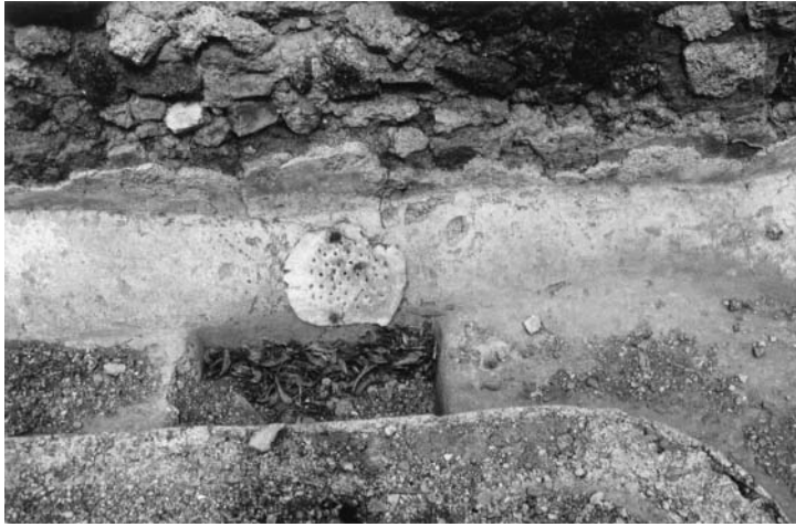
Figure 16.2 Settling box in peristyle gutter and perforated lead sheet in front of cistern entrance, both to prevent dirt from entering the cistern (Pompeii, I.9.11–12).
