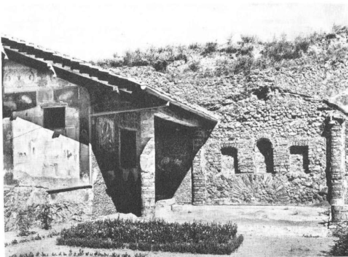
Figure 83 View of the nymphaeum and garden rooms at the House of Apolline (from an old photograph). The roof line of the nymphaeum can still be discerned in the bricks of the rear wall, whose three niches were designed to hold statues.
