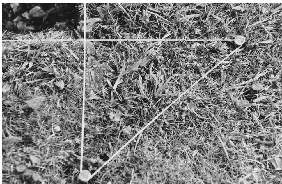
Figure 6.3 Stringing up the corner of a trench
