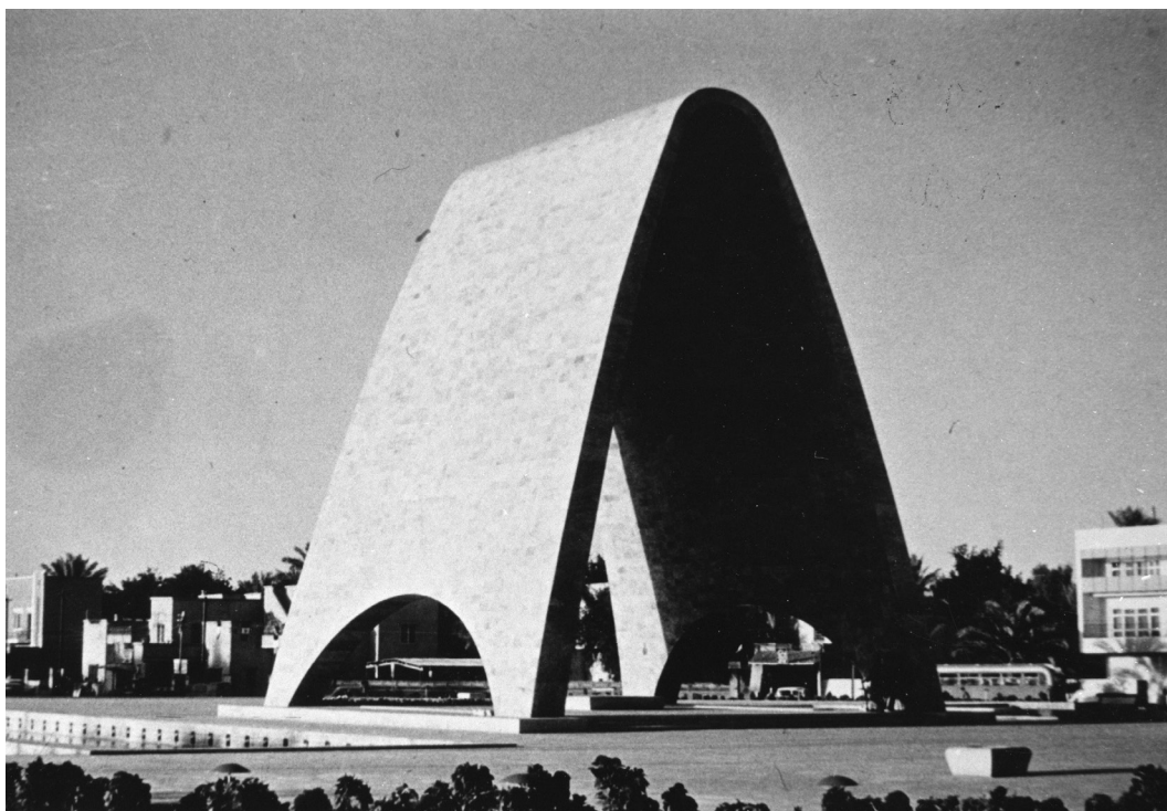
Figure 1: Photograph of Unknown Soldier Monument, Baghdad, 1959 (Kamil and Rifat Chadirji Photographic Archive). Courtesy of Aga Khan Documentation Center, MIT Libraries.
