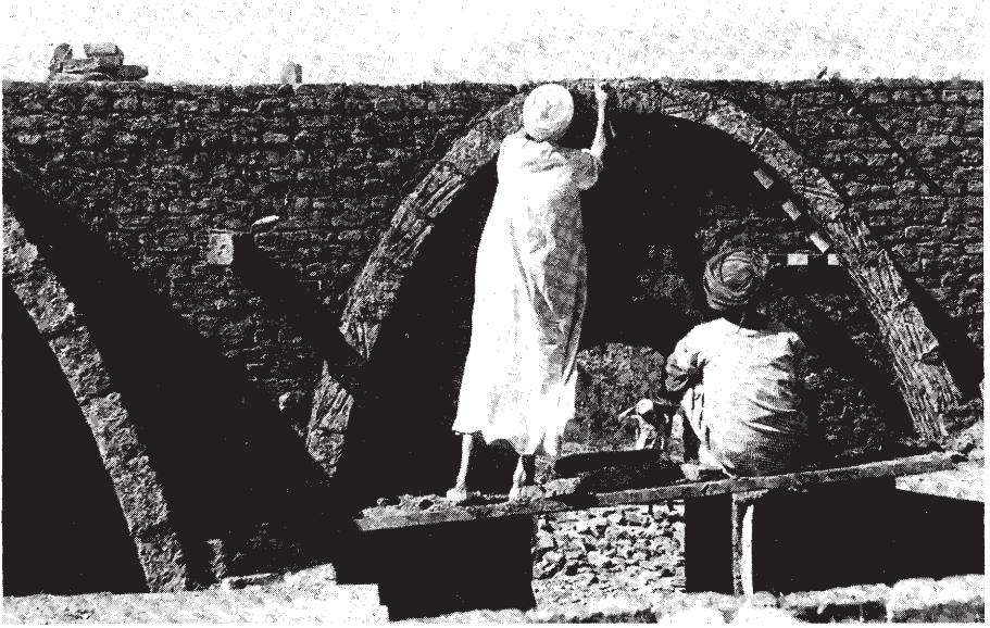
17. Masons insert dry packing in the interstices
