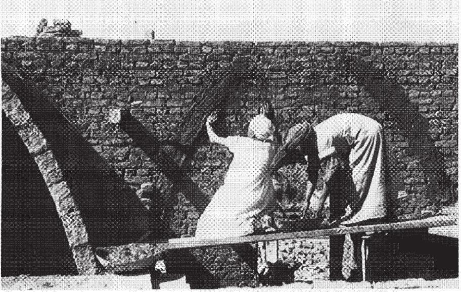
7. Masons outline a parabola on the end wall with mud plaster
