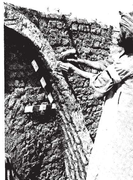
16. The first inclined ring is completed
