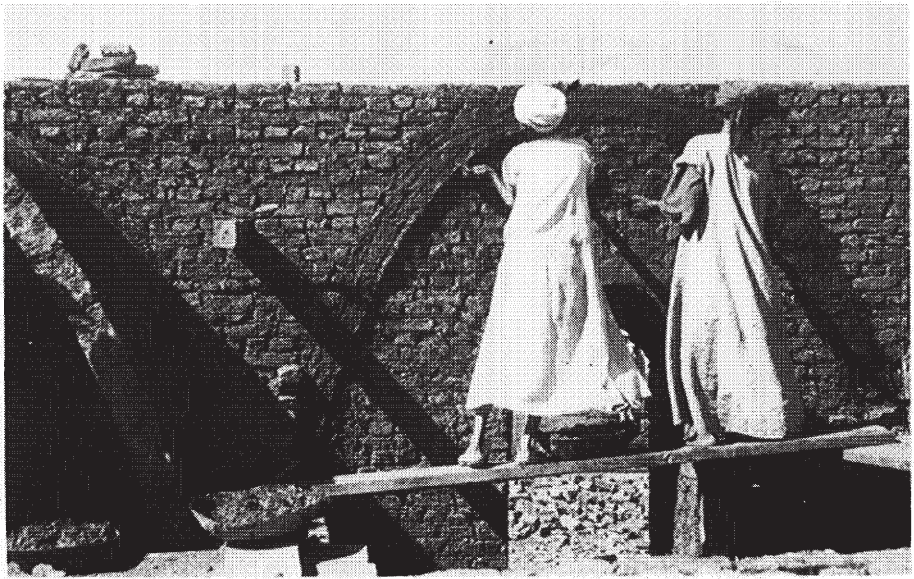
8. Trimming plaster with an adze
