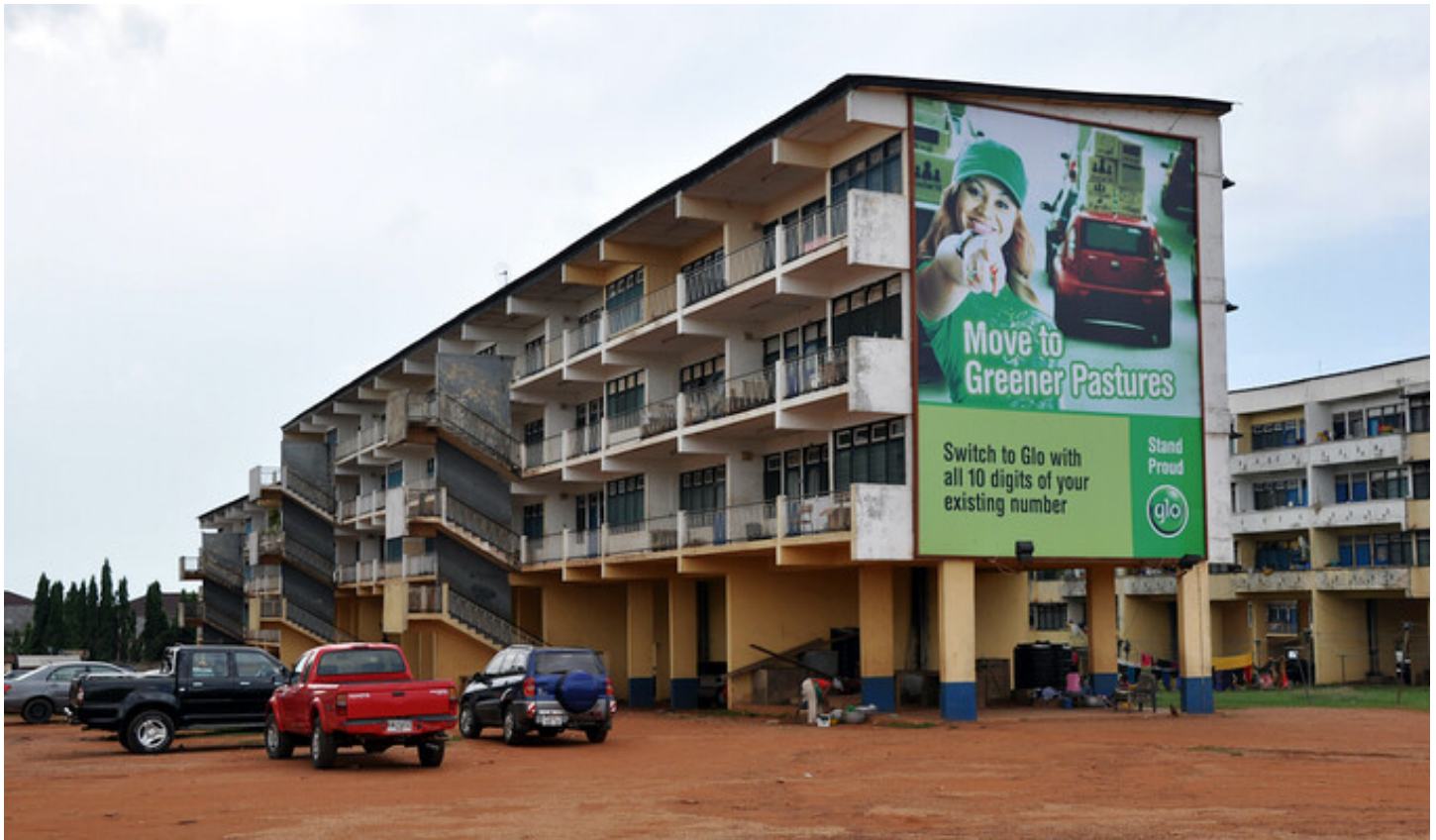
Flagstaff House housing project, Accra, 1964. Ghana National Construction Corporation, Vic Adegbite (chief architect), Charles Polónyi (project architect). Photo by Ł. Stanek, 2012. First published in: Stanek, Architecture in Global Socialism .
