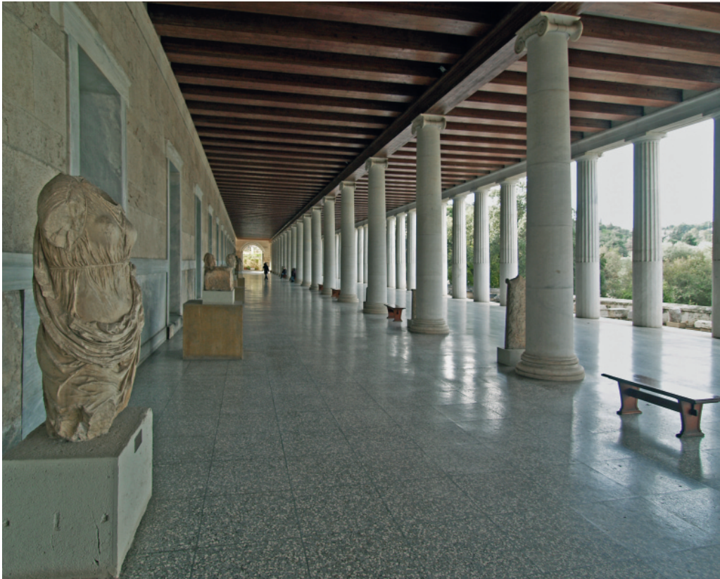
51. Lower colonnade from the Stoa of Attalos (Figure 50), ca. 150, rebuilt 1953–56. Large, arched openings at each end ventilate the two 20 ft. (6 m) wide promenades, and a central row of Ionic columns, unfluted like their Doric counterparts so as to minimize accidental damage, supports the ceiling and upper floor. Behind the columns, twenty-one shops and offices, each up to 16 ft. (5 m) square and almost 20 ft. (6 m) high, stretch the length of the building, echoed by another, less lofty set on the upper floor.
