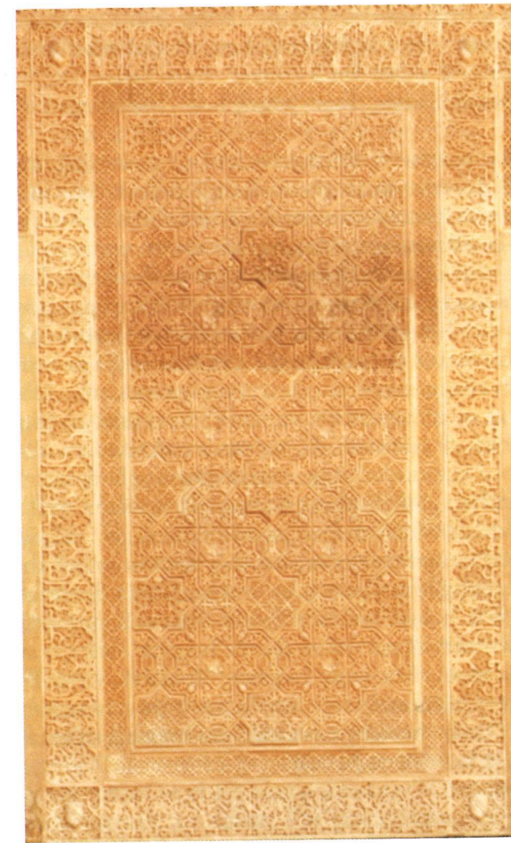
Figure 4.18 Façade of Comares, detail, central panel of carved stucco, Palace of Comares, Alhambra (photograph: Olga Bush)
