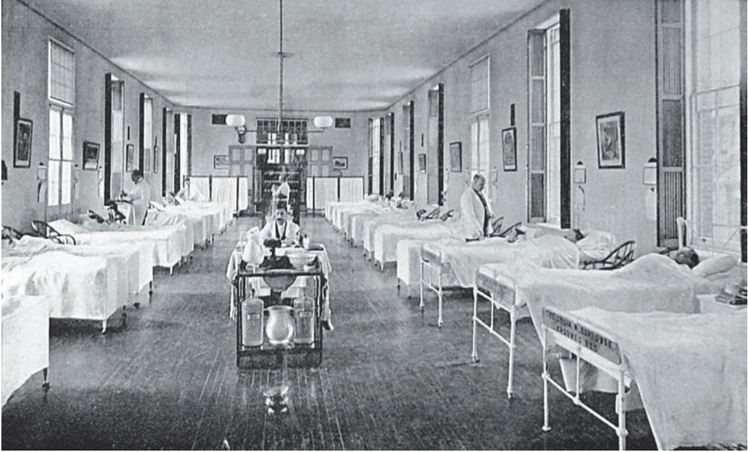
Figure 1.18. Roosevelt Hospital, New York City, view of male ward, 1893. Though a ward was one big open space, the windows determined bed placement both for air flow and maximum sunshine.
