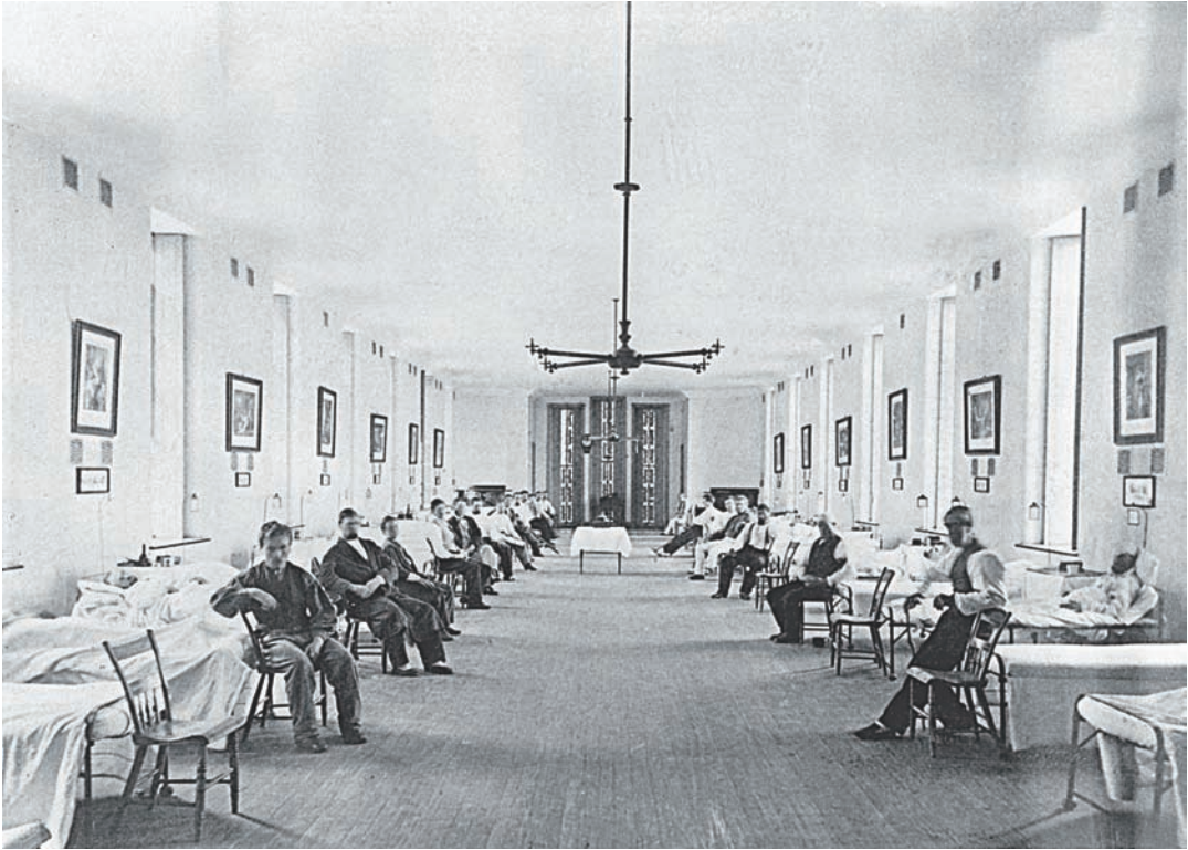
Figure 1.26. Hospital of the Protestant Episcopal Church in Philadelphia, view of male ward, 1869. Exhaust registers are visible on the wall just below the large pictures and close to the ceiling. There were also floor registers under the beds. All corners are rounded, all surfaces undecorated and seamless. The decorative treatment of the south-facing windows would have given the ward the ambience of a chapel, appropriate to the spiritual as well as physiological healing the founders intended to impart. The picture is posed to suggest that religious services are just about to start, the table in the middle of the ward serving as a makeshift altar.
