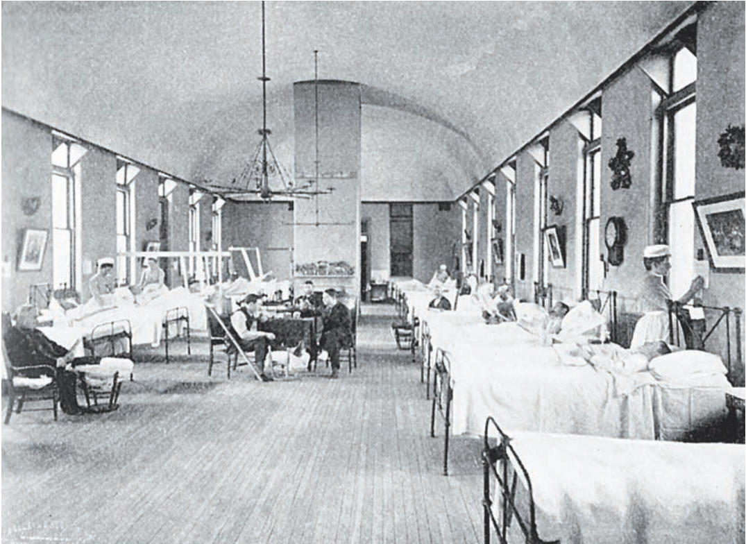
Figure 1.31. Bellevue Hospital, New York City, ward interior of Sturges Pavilion, 1893.
