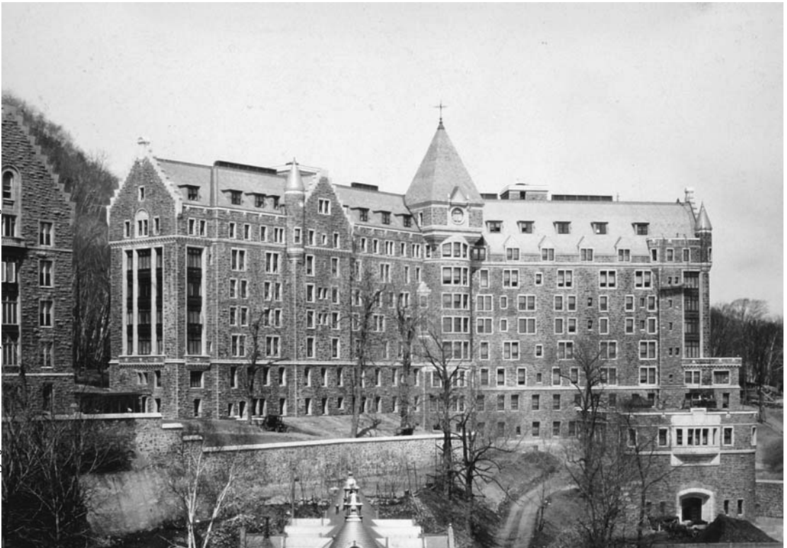
FIGURE 2.13. Royal Victoria Montreal Maternity Hospital.
