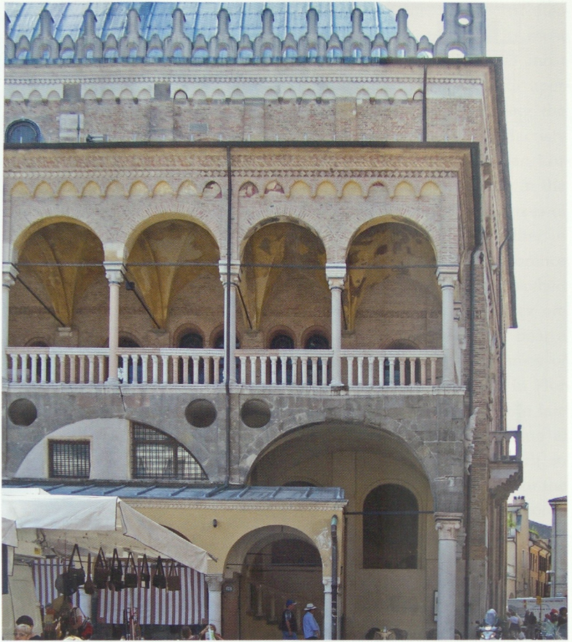
Fig. 25 Padua, Palazzo della Ragione, end-bays of the facade. The double-storey arcades (unknown architect) were added to the existing civic hall in the early 14th century (and the further arcade at the front was then attached subsequently).
