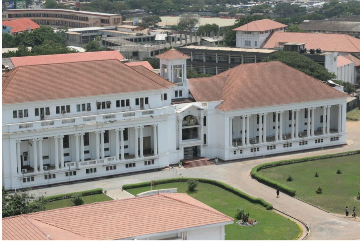
Supreme Court of Ghana in neoclassical style, construction started by the British in 1929
