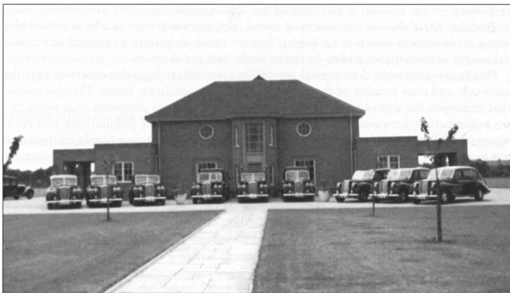
2.6 British crematoria are situated at the margins of society, in areas which are ambivalent in their landscape associations and meaning. Unlike churches which are often visited for aesthetic pleasure or spiritual contemplation, the interior of the architecturally undistinguished crematorium is seen only at funeral services.
