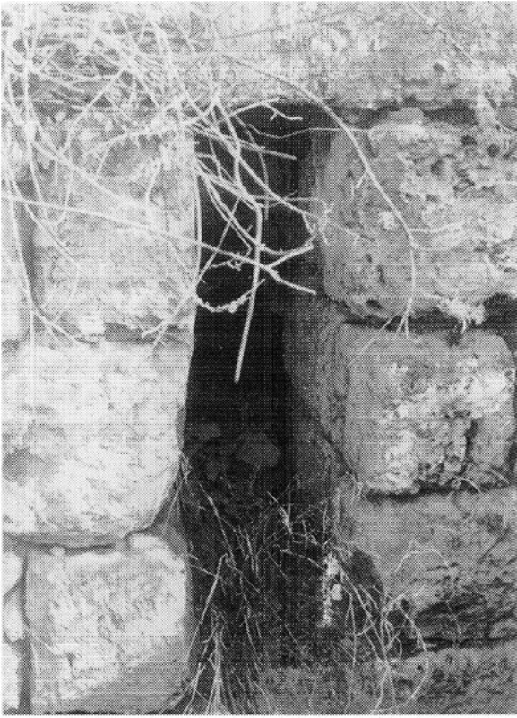
Figure 12.2. Slit in ramparts near the postern below the House of the Official, Morgantina. Such slits permitted runoff from inside the city to escape, possibly into an irrigation system outside, rather than build up behind the walls and endanger their stability. The slit is too small for anyone but a small child to penetrate, being approximately .3 by .6 meters.
