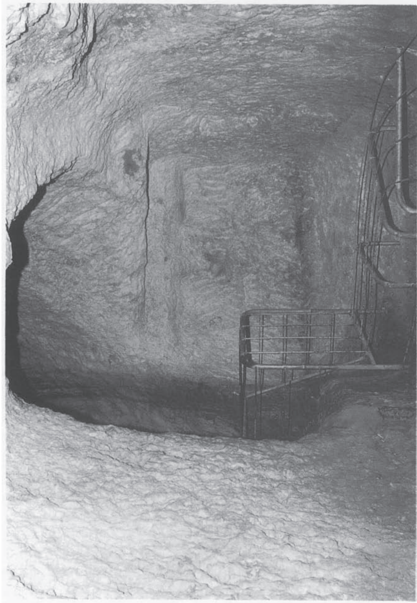
Figure 18.3 The junction—the abandoned face of the south tunnel is straight ahead, and the north tunnel joins at left.
