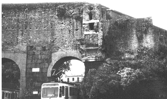
Fig. 8.4: A pier of the Aqua Marcia preserved in the later Aurelian Wall. The smaller channels of the Tepula and Iulia are visible above the stone channel of the Marcia (Photo: author).
