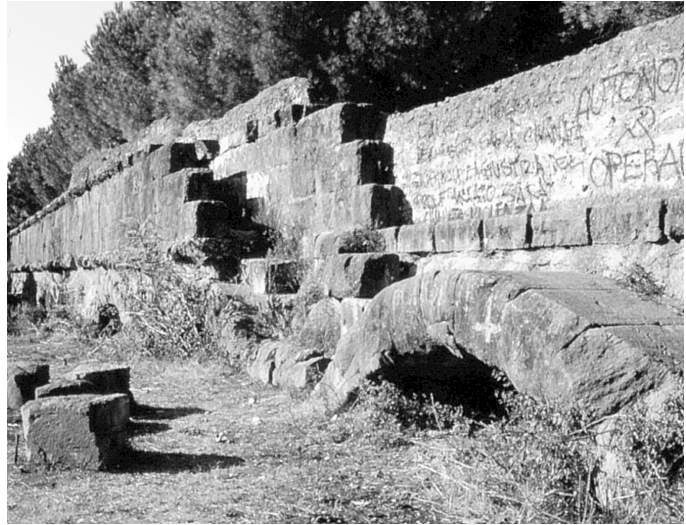
Fig. 8.3: The channel and arcade of the Aqua Marcia at Romavecchia. The channel of the Aqua Tepula partially survives on top (Photo: author).
