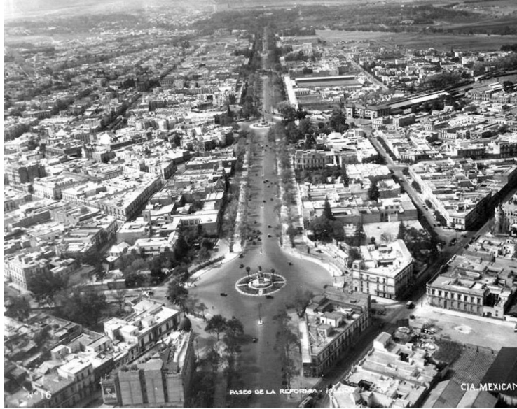
Paseo Reforma, a large boulevard expanded and remodeled in the image of Haussmann's Paris, c. 1880–1910
