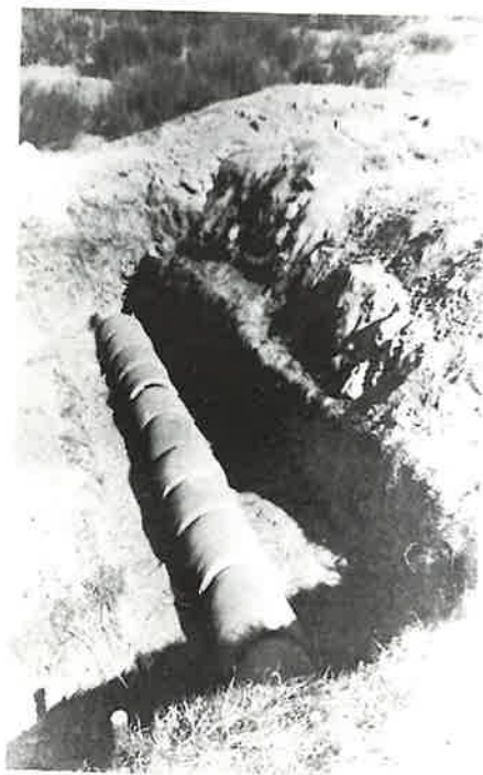
70. Mt Beuvray, France: pipeline made of re-used amphorae, with tops and bottoms removed so that they fit into each other. Photograph by the excavator, J. Délechette, in 1907 (photo © Beuvray).
