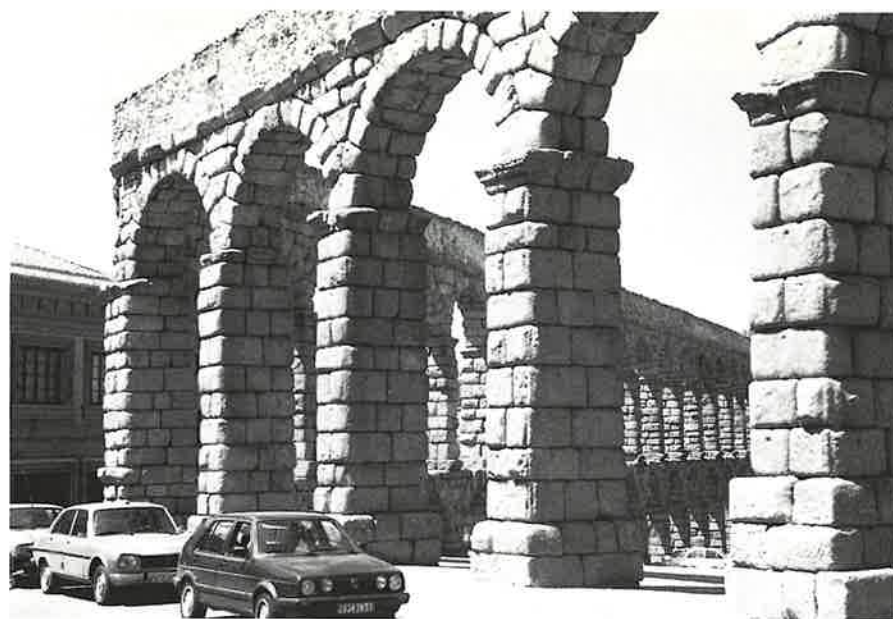
73. Segovia: angle in the arcade. There are no buttresses to counter centrifugal force at the bend.
