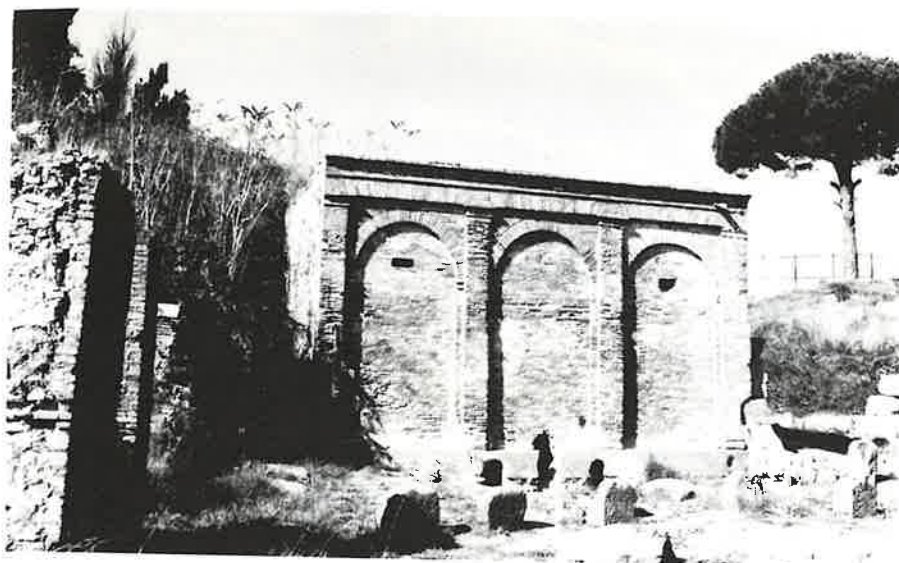
196. Pompeii: castellum divisorium , at the Porta Vesuvii. Plan of the interior arrangements, Fig. 197. Water mains serving the city came from the three large openings at the base of the wall.
