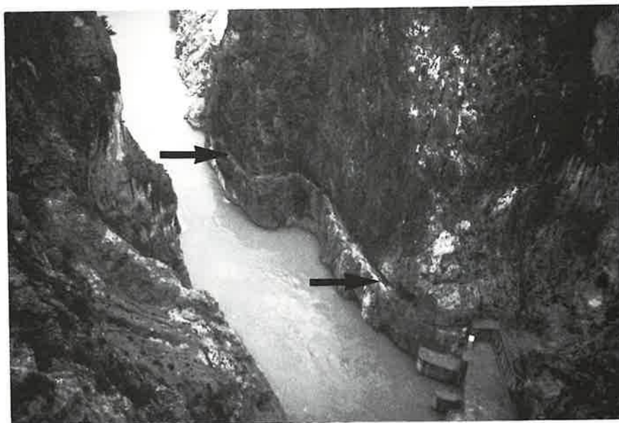
59. Side, Turkey: rock-cut channel carrying the Roman aqueduct (indicated by arrows) along the gorge of the river Manavgat, immediately below the modern dam.
