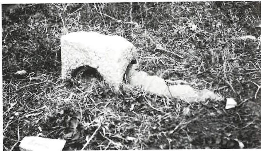
72. Miletos: stone angle block in situ at bend on terracotta pipeline.
