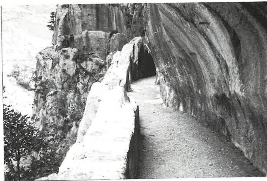
58. Side, Turkey: rock-cut channel of the aqueduct (photo: H. Fahlbusch).
