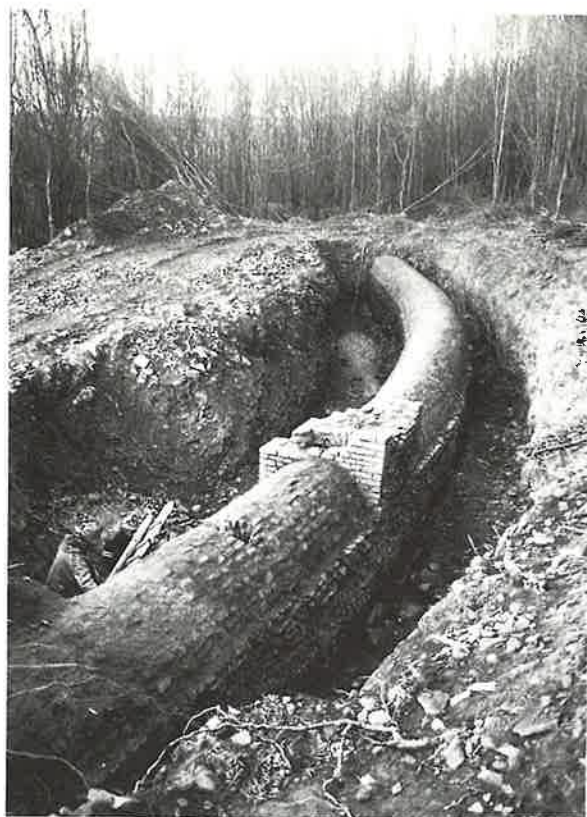
46. Cologne, Germany: a stretch of the Eifel aqueduct, showing vaulted roof and an inspection manhole; normally subterranean, this section was uncovered during road-building (photo: K. Grewe, Bonn).
