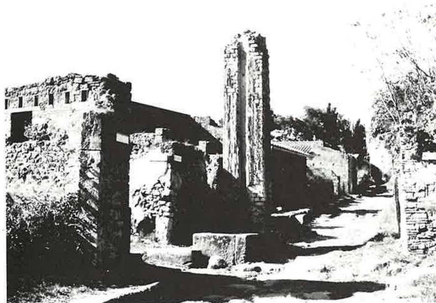
204. Pompeii: water tower. Clearly visible are the vertical recess carrying the piping up its side to the tank on top, and the public fountain (the square stone basin) at its base.
