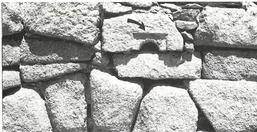
63. Segovia: re-used block from a stone pressure pipeline (arrow) embedded in the arches of the Roman aqueduct.
