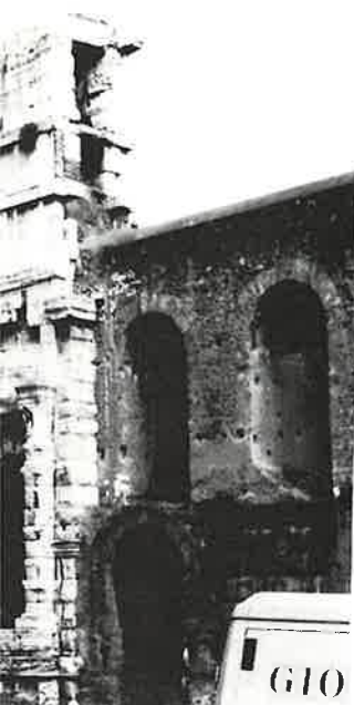
Porta Maggiore, the point at which the eastern aqueducts entered Rome. The channels of the Aqua Claudia and the Anio Novus are clearly to be seen on top of the walls.
