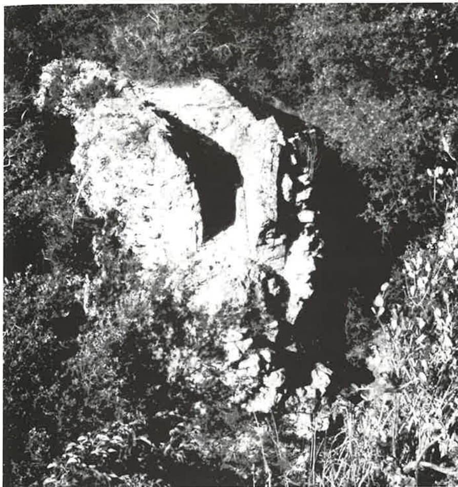
47. Pont du Gard: the conduit of the Nimes aqueduct, a short distance to the south of the great bridge. The channel, here running at ground level, has lost its vaulted covering but clearly shows the thick sinter incrustation on its sidewalls.
