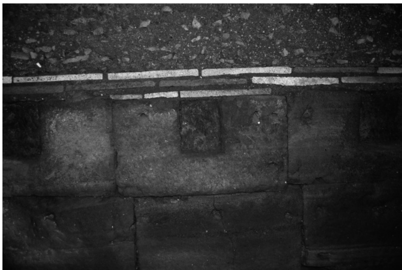
5.7 Cloaca Maxima. Detail of Augustan tufo and Domitianic concrete under Forum Transitorium. Photo: John Hopkins.
