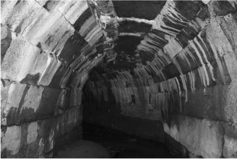
5.5 Cloaca Maxima. Domitianic tract east of temple of Minerva in lapis Albanus. Photo: John Hopkins.
