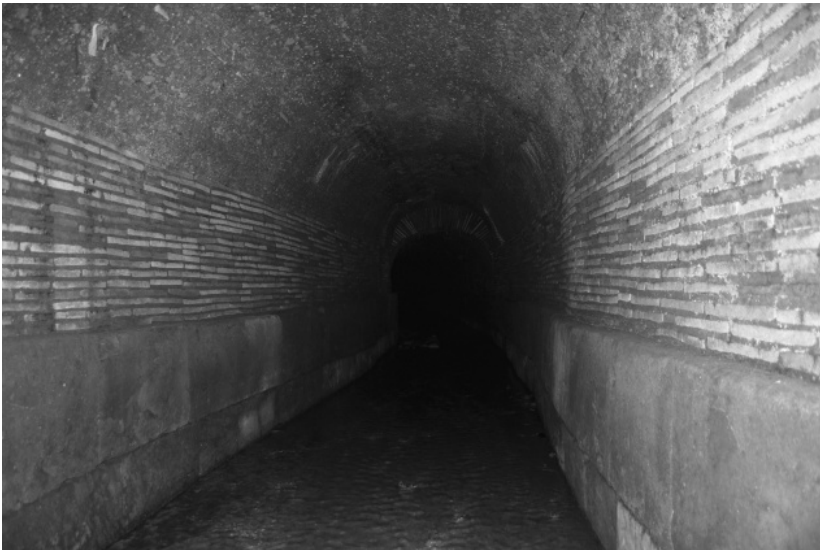
5.6 Cloaca Maxima. Augustan tract under Forum Transitorium in lapis Gabinus with Domitianic concrete vault. Photo: John Hopkins.
