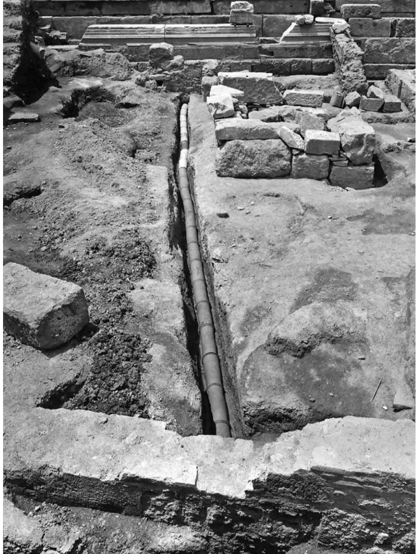
Figure 20. Early pipeline from the northern overflow channel of the Southeast Fountain House, in situ. Shear 1935, p. 335, fig. 22; courtesy American School of Classical Studies at Athens
