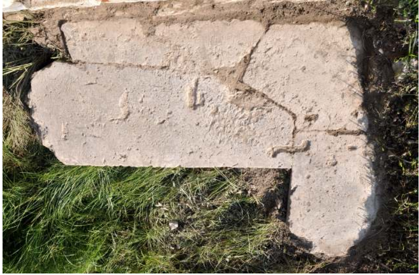
Figure 3. Detail of northeast corner of Southeast Fountain House showing Z-clamp cutting. Photo J. Paga
