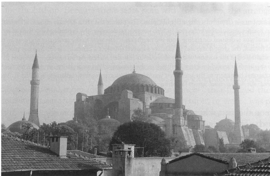
Fig. 4.2 Constantinople (Istanbul), Hagia Sophia, general view from the southeast. The cascading forms of the high vaults are evident at the east and west ends: the hemispherical dome is braced along the main axis by half-domes, which in turn are braced by the conches of niches. (R. Ousterhout)
