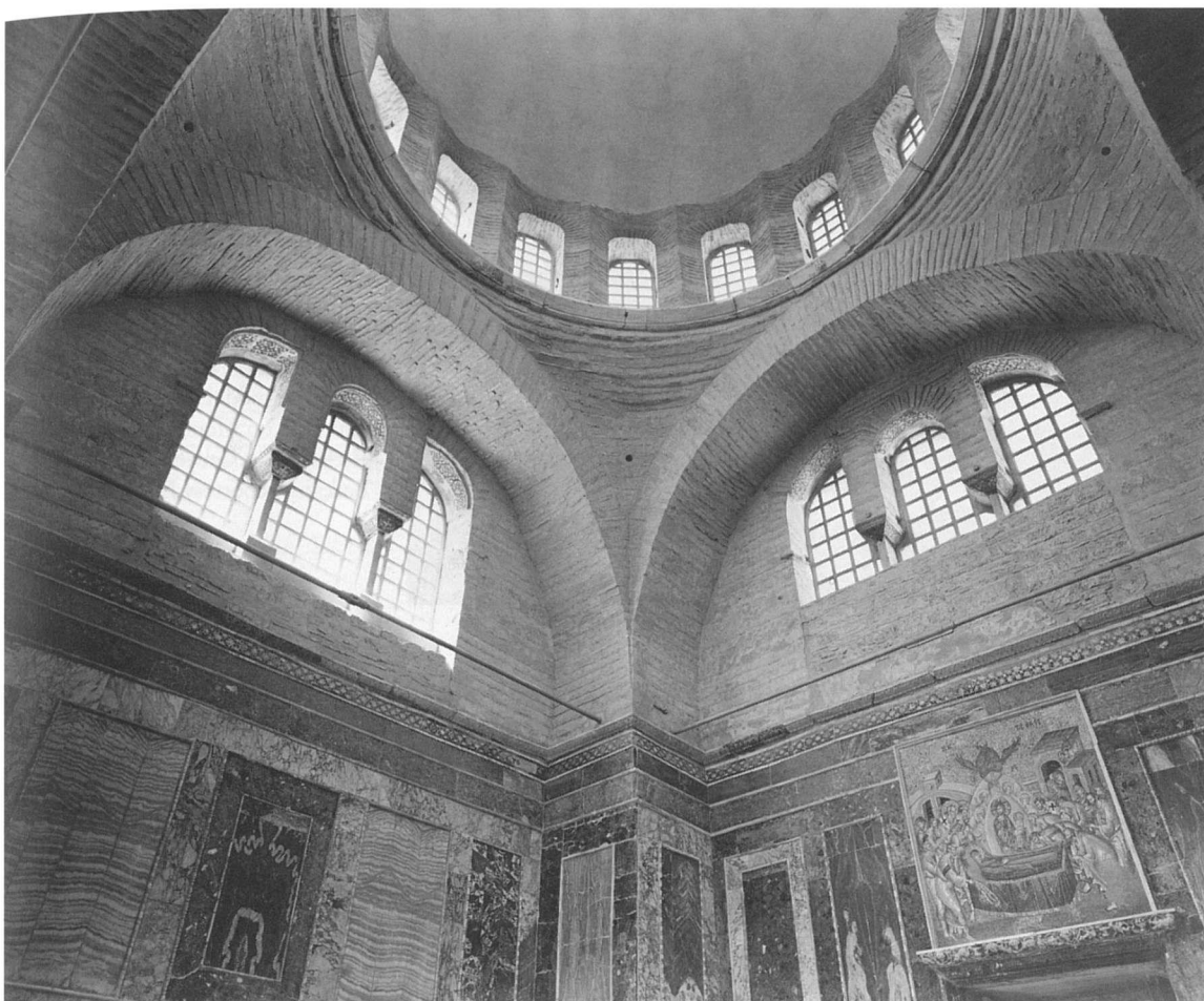
Fig. 4.24 Constantinople (Istanbul), Chora monastery, interior of the twelfth-century naos. Four narrow arches rise from the corner piers to support the dome, creating a unified interior and opening large wall areas in the lunettes for windows. The dome was rebuilt in the fourteenth century. (courtesy Dumbarton Oaks)
