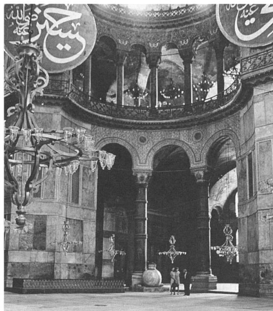
Fig. 4.9 Constantinople (Istanbul), Hagia Sophia, interior, detail of exedra. The colonnaded niches at each corner of the nave create a billowing effect that helps relate the main space to the ancillary spaces. The gallery colonnades are not aligned with those on the ground floor: this counteracts their structural potential and emphasizes their decorative role. The great roundels flanking the exedra are inscribed with Muslim prayers and are remnants of the Ottoman period. (T. Mathews, courtesy Dumbarton Oaks)
