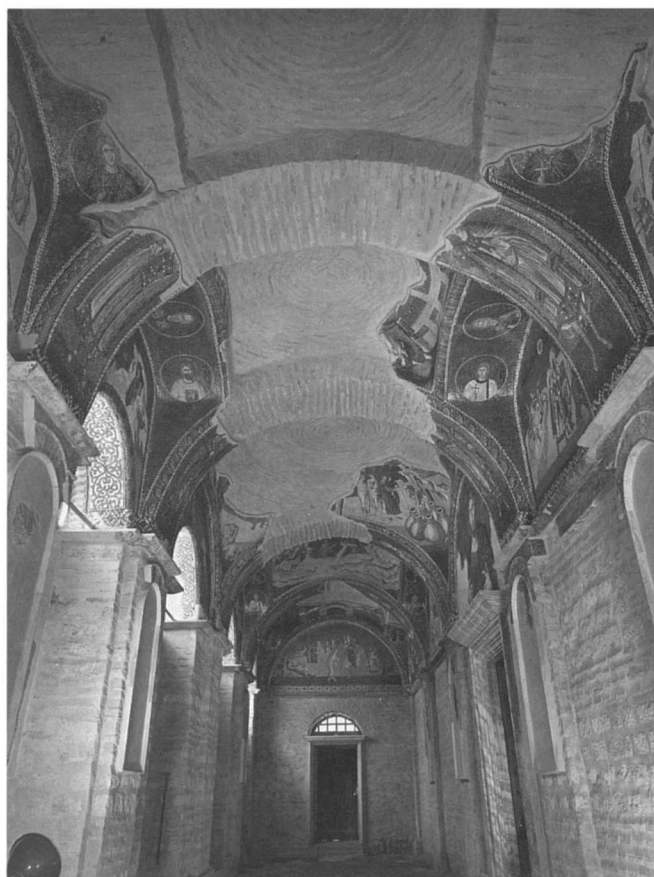
Fig. 4.41 Constantinople (Istanbul), Chora monastery, interior, view of exonarthex looking north. The curious vaults have arches springing from arches to create a square that could be covered by a sail vault, in which the pendentives are extended to form a continuous curve. The vaults provided surfaces for narrative scenes in mosaic, whereas the arches were decorated with images of saints, organized according to the liturgical calendar. (courtesy Dumbarton Oaks)
