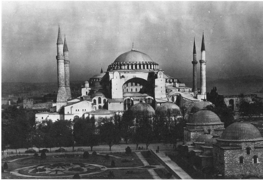
Fig. 4.1 Constantinople (Istanbul), Hagia Sophia, general view from the south. The centrally positioned dome is the dominant element in the innovative design of Justinian's "Great Church," with lower half-domes to the east and west. Clerestory windows filled the lunettes, the semicircular walls to the north and south. The large buttresses were part of the original construction, meant to stabilize the high vaults of the church. Numerous accretions, including the adjacent tomb buildings and the minarets, were added during the Ottoman period when the building functioned as a mosque. (courtesy Dumbarton Oaks)
