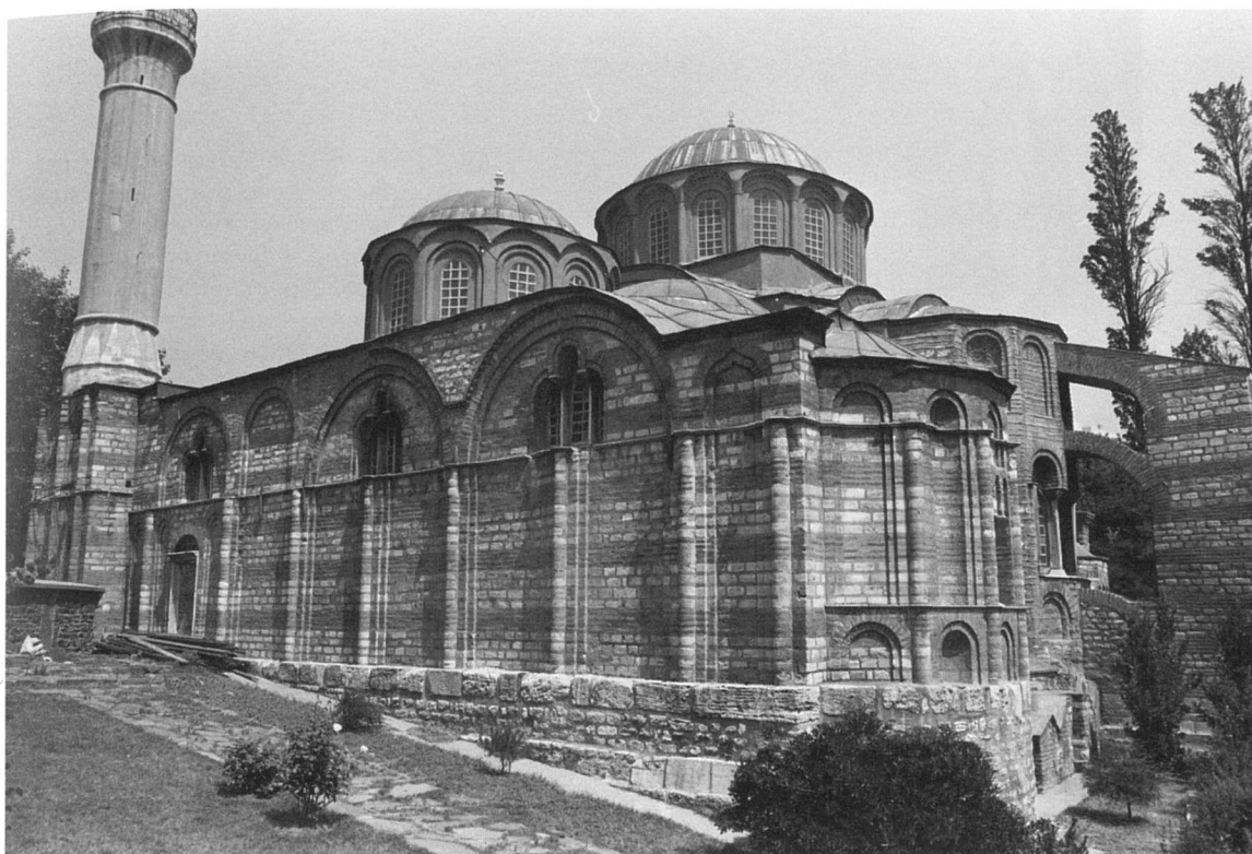
Fig. 4.39 Constantinople (Istanbul), Chora monastery, general view from the southeast. The facades are enlivened by niches, pilasters, and engaged columns. To the east, a flying buttress—one of the few in Byzantine architecture—braces the apse on unstable terrain. Along the south facade, the rhythm of supports is quickened, and stepped responds (pilasters behind a column) and half-columns appear to be illogically “supporting” windows. Taken out of their structural role, they become part of the manneristic decoration of the church. (R. Ousterhout)
